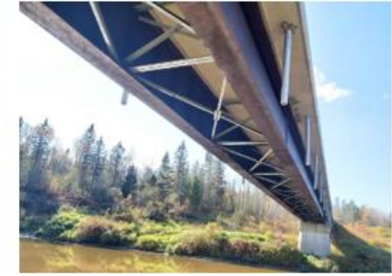
Photo 2: Central Span (looking east)
