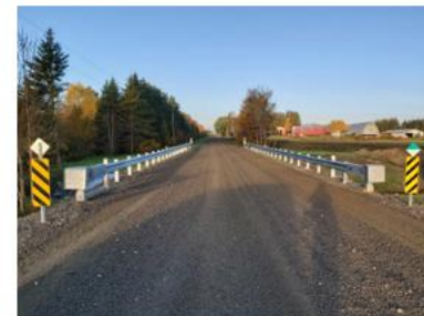
Photo 4: East Approach (looking west)
