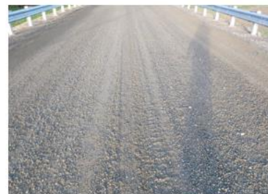
Photo 5: Wearing Surface (looking west)
