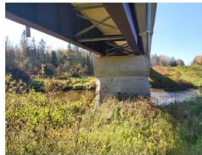
Photo 3: West Pier (looking east)
