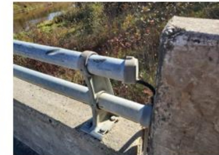
Photo 6: Bell line Run Through Railing
