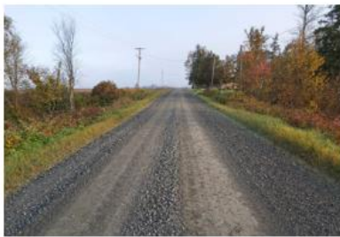
Photo 4: South Approach (looking north)
