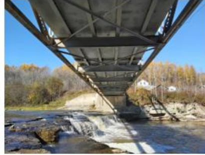
Photo 2: Structure Soffit (looking west)
