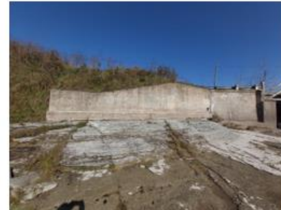
Photo 6: Northwest Retaining Wall
