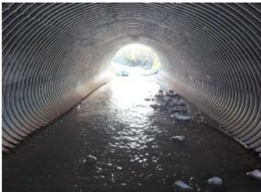
Photo 3: Inside Barrel (looking east)
