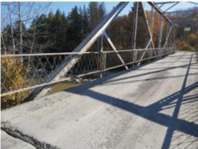
Photo 3: South Railing (looking west)
