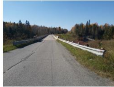
Photo 1: East Approach (looking west)
