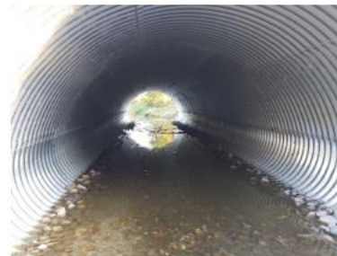
Photo 3: Inside Barrel (looking north)
