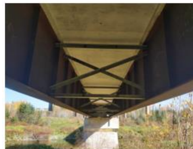
Photo 5: East Span (looking west)
