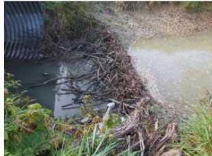
Photo 6: Beaver Dam at Upstream Inlet
