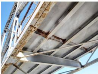
Photo 5: Corrosion on Floor Beam Braces
